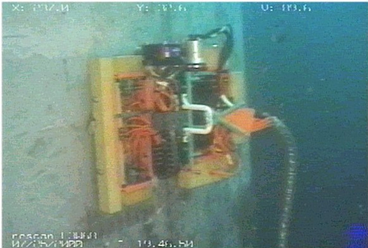
ROV version of AUS-4 performing weld inspection on platform leg
